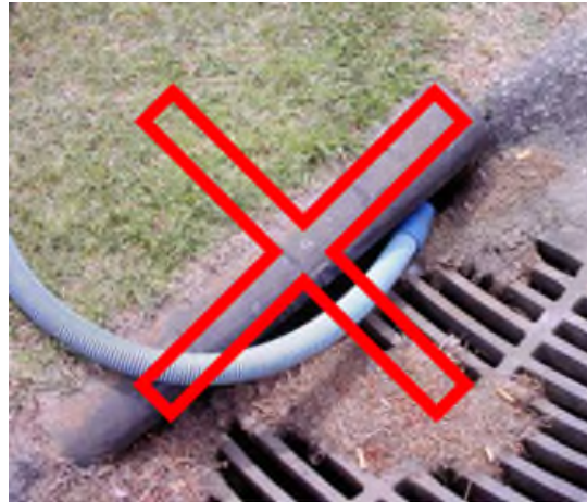
Figure 13 Improper Discharge of Pool Wastewater
