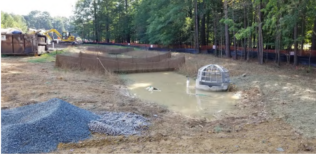
Figure 11 Example of Construction Site Runoff Controls: silt fence, sediment pond
